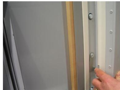
2. Unscrew the screws and open the inner door to reach the lock area
